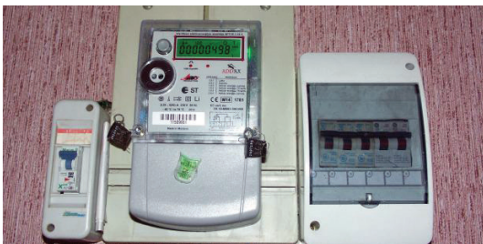
Fig. 5.3. A smart meter used by AS Sadales tīkls.
