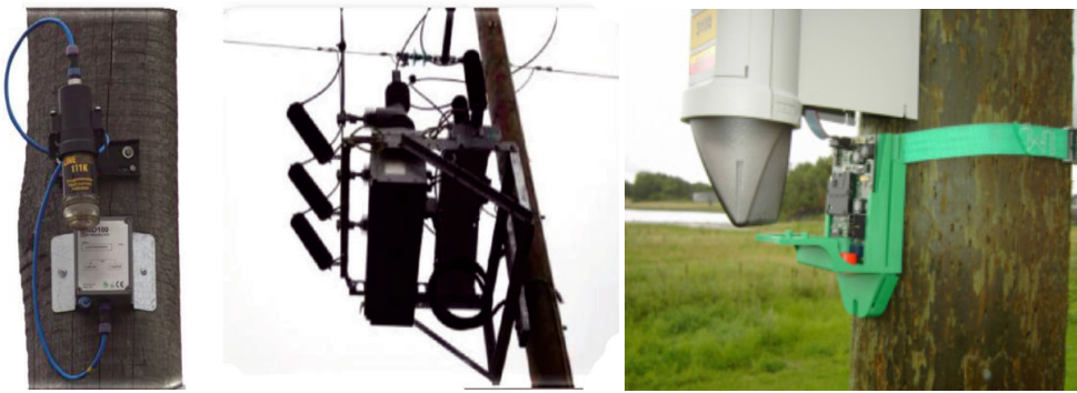
Fig. 5.5. Damage indicators used by AS Sadales tīkls [27].
