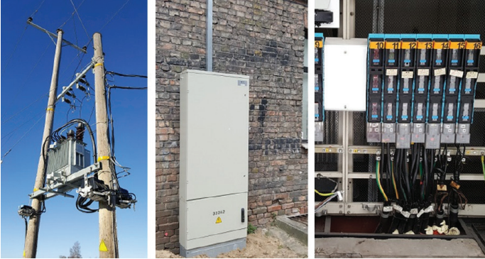
Fig. 4.7. New electrical installations in distribution network following reconstructions.
