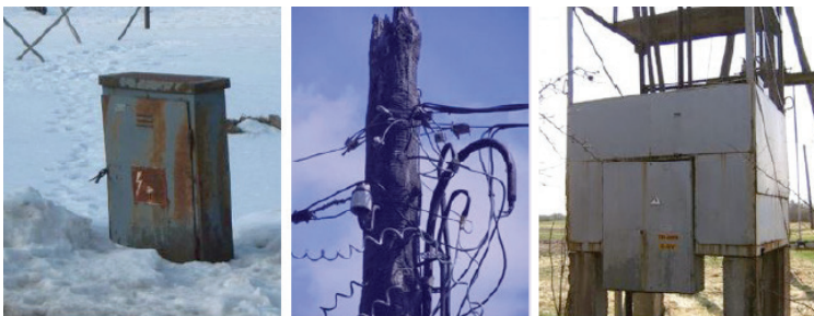
Fig. 4.6. Worn electrical installations in distribution network objects.
